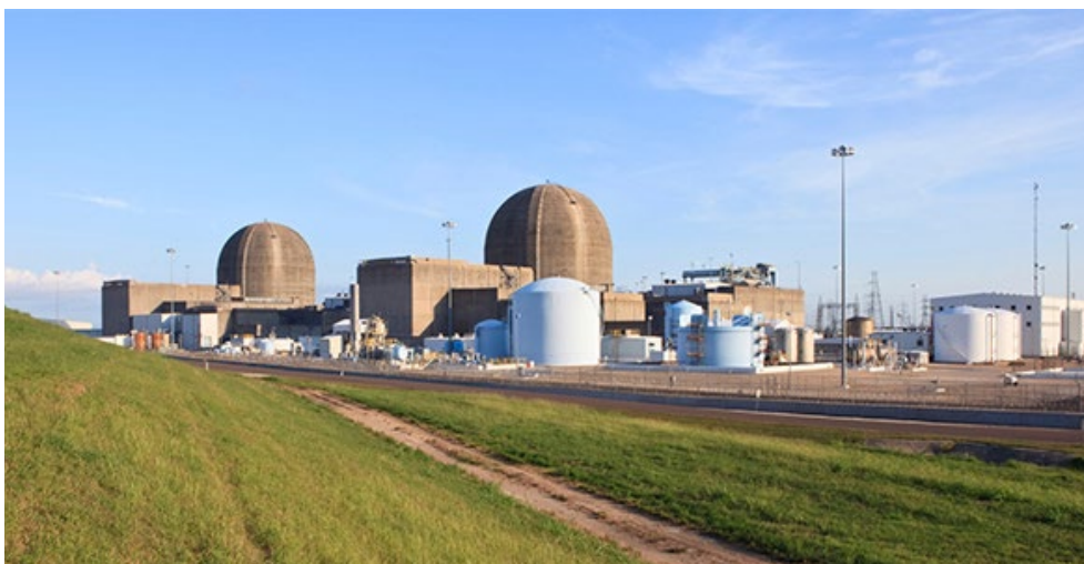
The South Texas nuclear plant suffered an outage from Feb. 15 to 17 because of a frozen pressure sensor line, which caused water pumps to trip. | NRG
